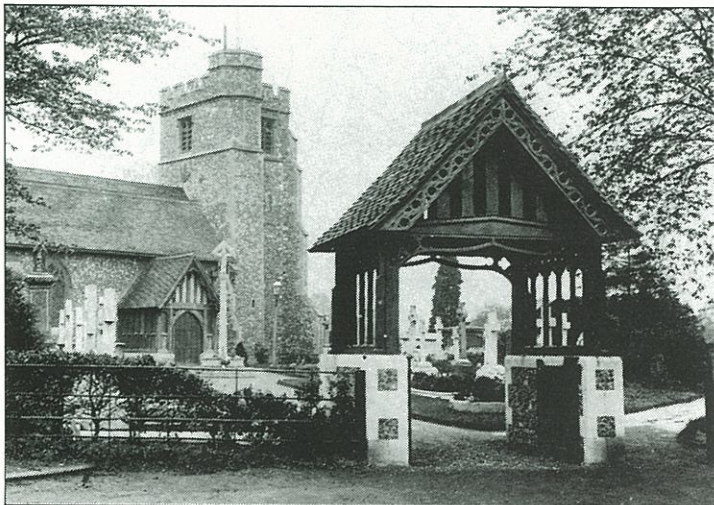
Bushey's ancient parish church of St James is reputed to have been founded in 1006. The Lych Gate was erected to commemorate those who died in the 1914-18 War; it was destroyed by a stray bomb in the 1939-45 War.
