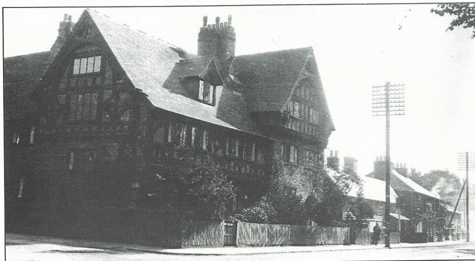
[Below] The Bavarian-style house built by Herkomer, pictured early this century. The furthest half then housed Bushey College. (see article opposite)
