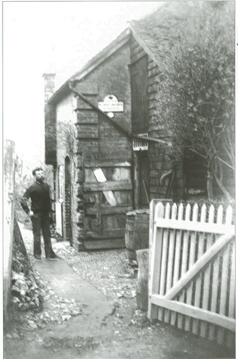
Police horse patrol station in the Bushey area. The location is not Church View where Bushey's police station was originally based, but possibly Aldenham.
