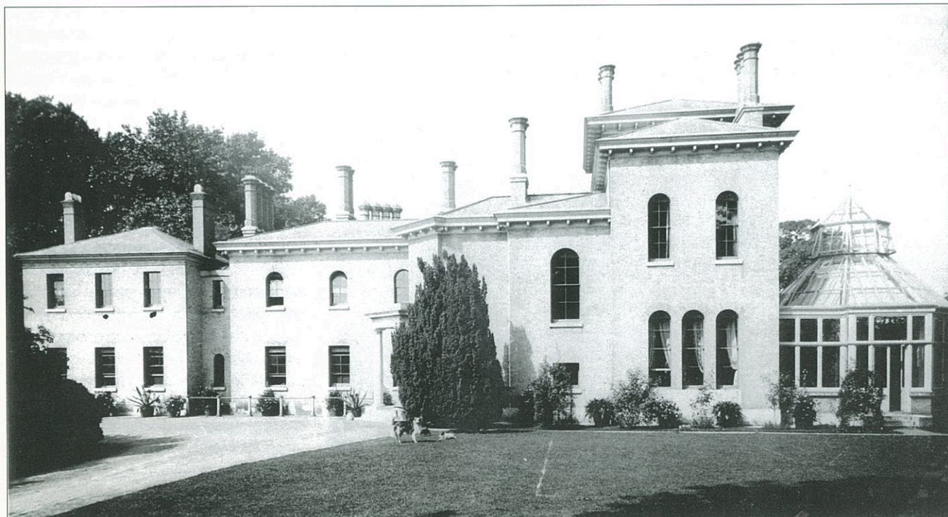
The front of Haydon Hill House in Merry Hill Road in about 1910.
