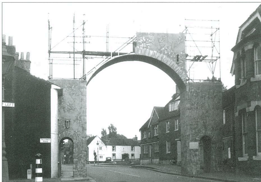
The 1953 Coronation Arch under construction. It was made of scaffolding and plywood but there were protests when it was dismantled six months later.
